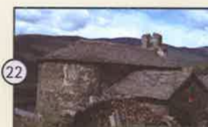
22 Sant Joan d'Avellanet: A small Romanesque church built in the late 11th century, it is one of the main examples of this style in the Pallers valley.
