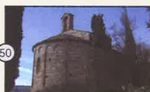
50 Sant Miquel de Peramola: The church of the cemetery of Peramola built in the 11th century. Only the apse is preserved from the original Romanesque building. The rest of the building is the outcome of a curious historicist reform.
